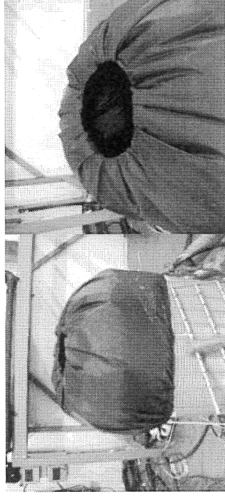
Figure 2. An Example of a Condenser Air Exit Restrictor
