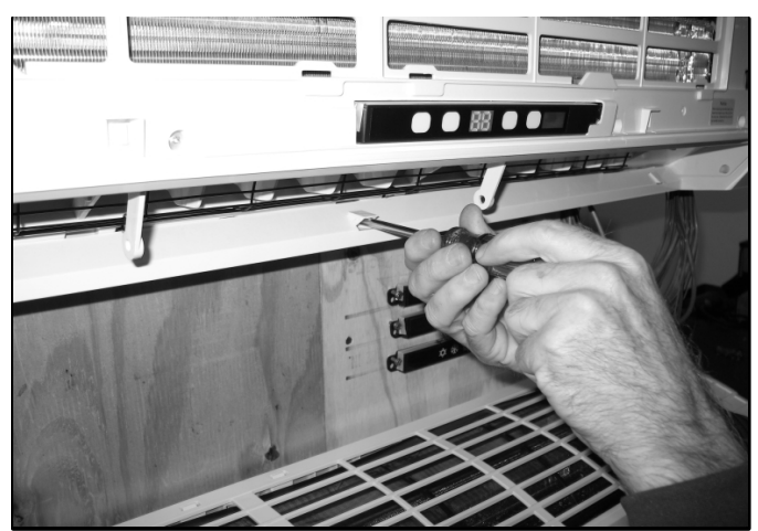
4. Remove the screw(s) that secure the indoor terminal strip access cover.
