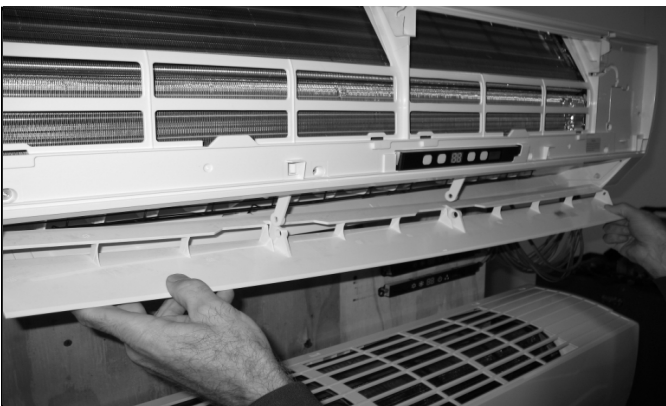
4. Remove the screw(s) that secure the indoor terminal strip access cover.
