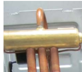
REVERSING VALVE BODY
