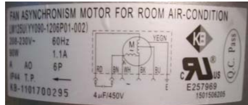
PHOTO OF OUTDOOR FAN MOTOR NAME PLATE (18-24 KBTU UNITS)
