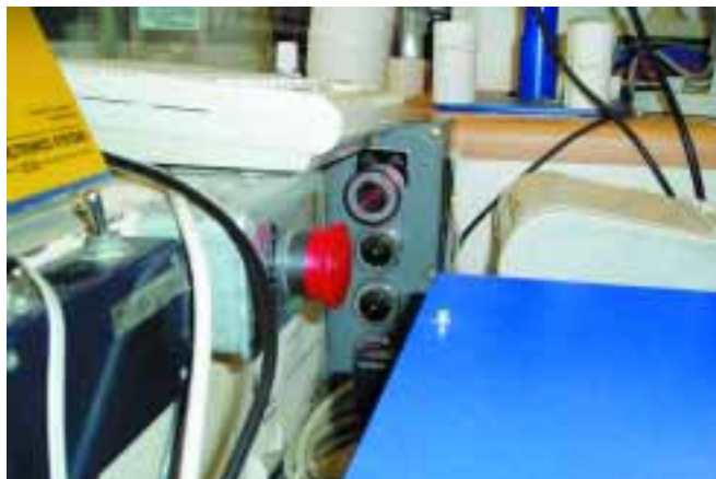
The spill incident was made worse because the emergency shut-off switch was partially hidden.
