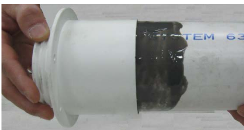
Assemble while cement is wet & soft
