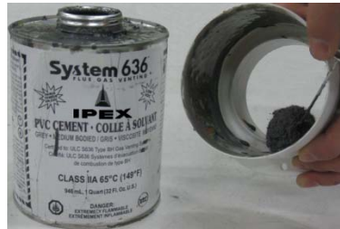
Cement Interior of Navien collar (socket)
