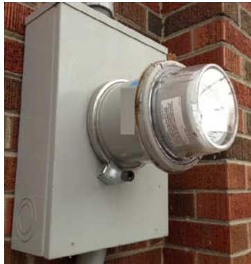
Photo B1 - External Load Limiter
