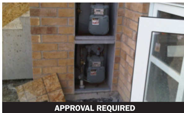
Figure 4: Stacked Meter Boxes - Approval from Enbridge Gas Distribution is required during the architectural design stage prior to installation.
